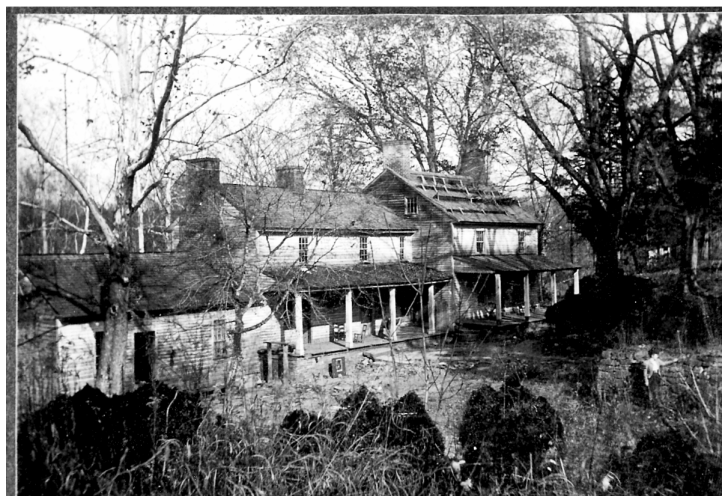
James Mendenhall House demolished 1928. Courtesy High Point Historical Museum
